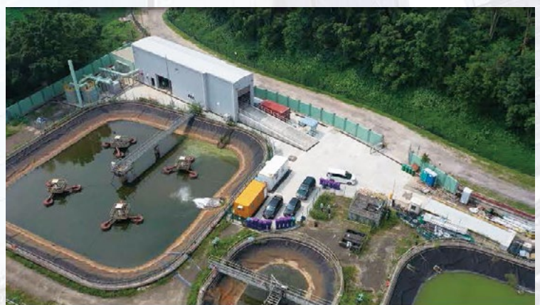
Food waste – sewage sludge anaerobic co-digestion in Tai Po STW
