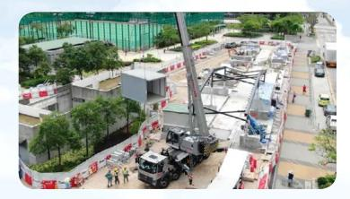
Modules of the MiC containers for market stalls were manufactured off-site and transported to site for assembly
